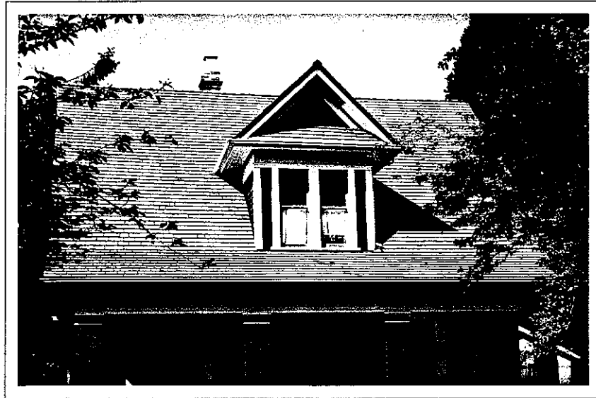
Dormer facing street breaks up large sloped roof
