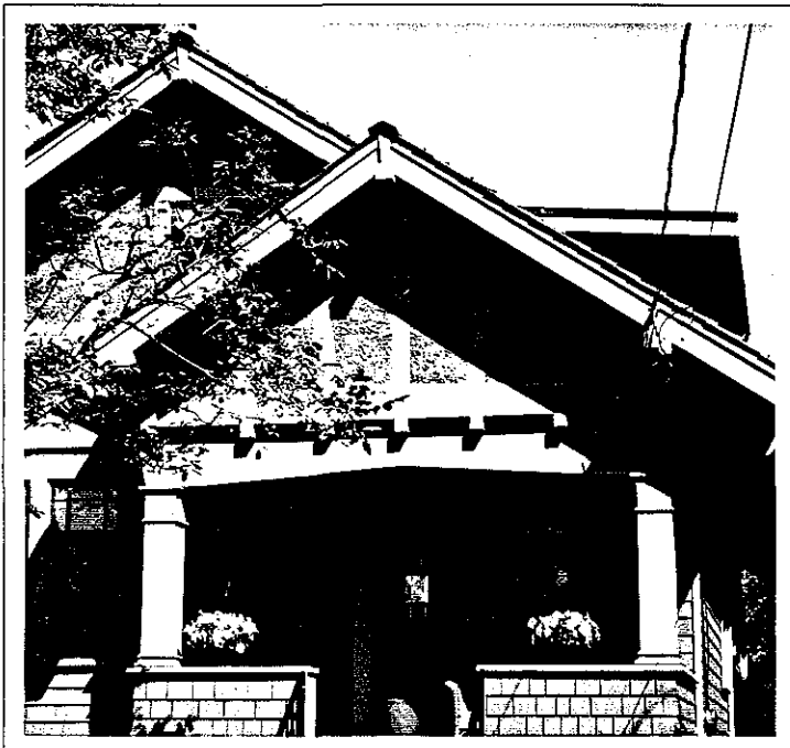
Stucco used as infill material
