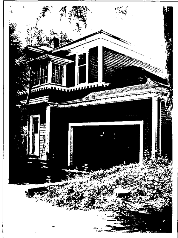
New garage addition compliments house
