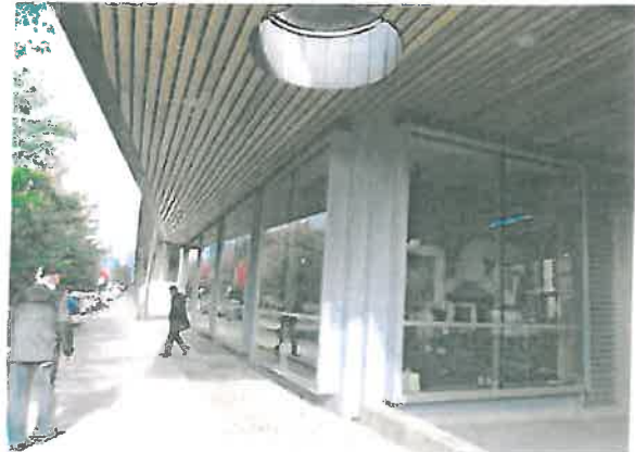
Vancouver’s False Creek Sewer Heat Recovery
