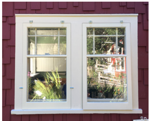
Exterior storm windows can improve the performance of original wood windows. Source: Vintage Woodworks
