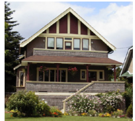
Porches were designed to cool exterior walls, allow windows to be opened all year long and provide a sheltered living space.
