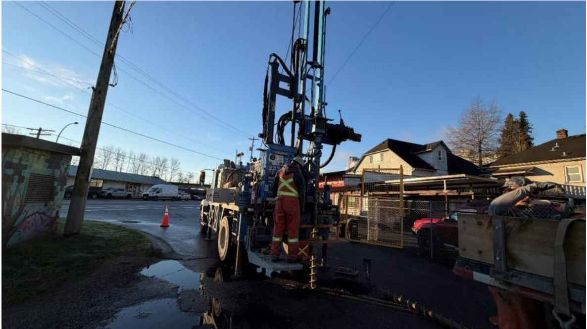
Photograph No. 1 Drilling in progress at AH26-01; photograph taken facing west. Dated 15 January 2026.
