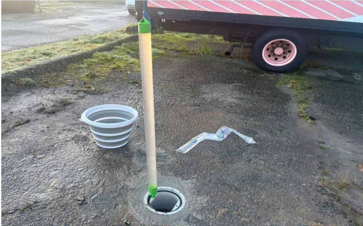
Photograph No. 7 View of groundwater well development at AH26-02. Dated 16 January 2026.
