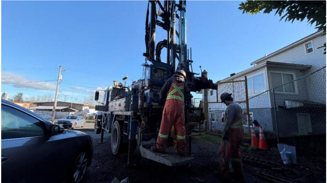
Photograph No. 3 Drilling in progress at AH26-03; photo taken facing north. Dated 15 January 2026.
