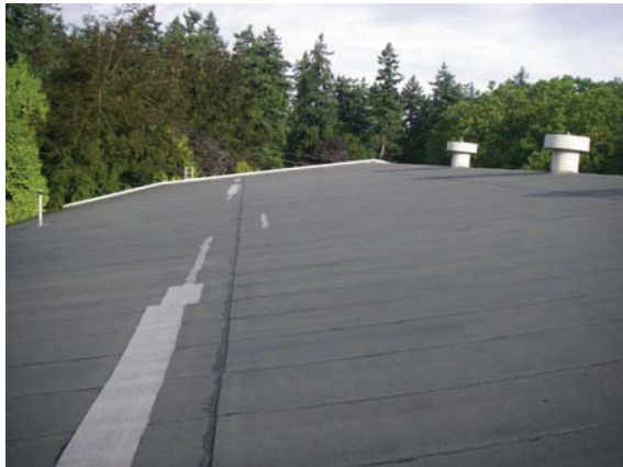
West side of roof
