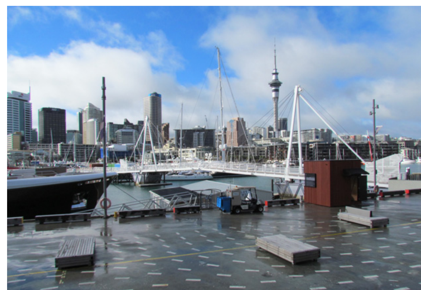
Example of a bascule bridge in Auckland, New Zealand
