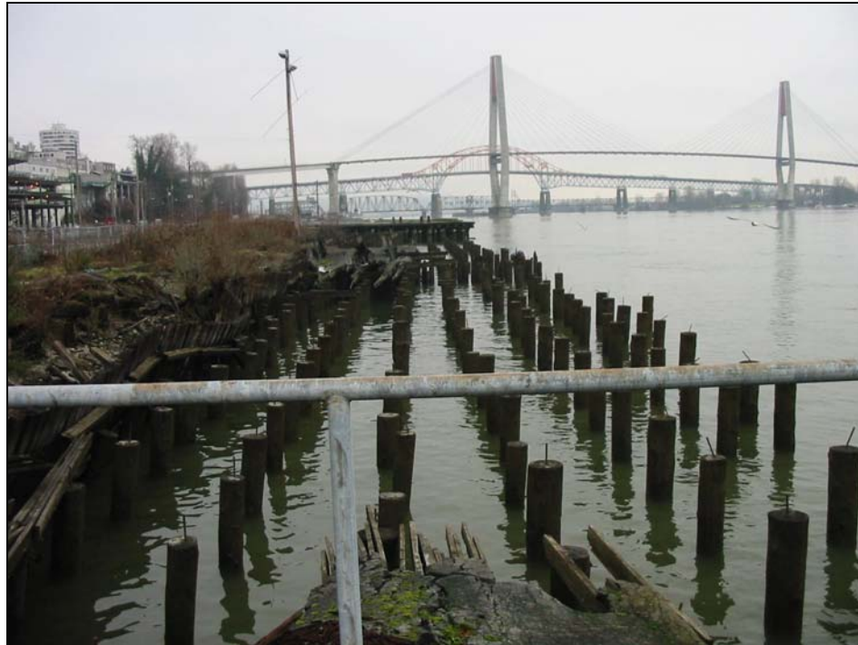
Photograph 3: A section of the wharf toward the southeast of the Site
