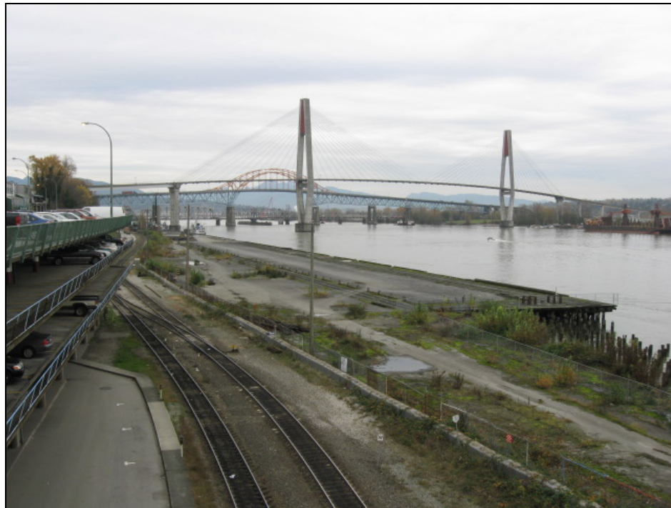
Photograph 2: Another view of the Site, facing east
