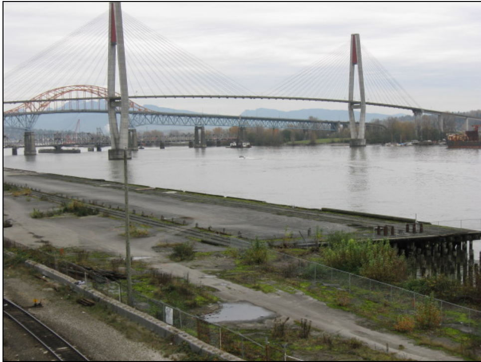
Photograph 1: A view of the Site, facing east
